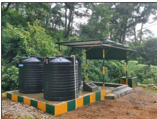
Water Conservation Cum Distribution Work
