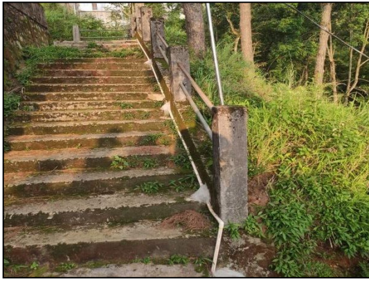
CPVC Distribution Pipeline
