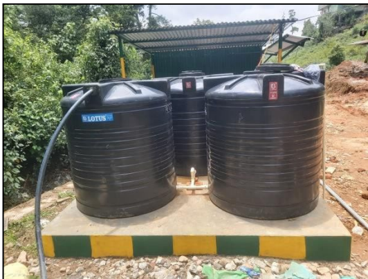
Water Storage Tank
