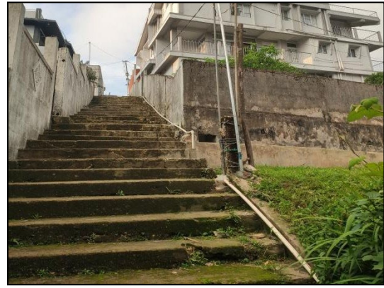
CPVC Distribution Pipeline
